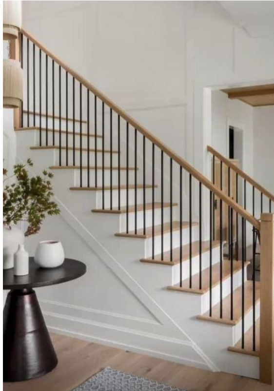
Black Round Iron Spindles w/ Contemporary White Oak Newels and Handrail.
