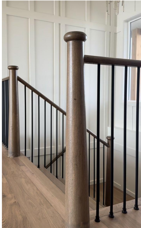
Wood Handrail and Newels & Black Iron Round Spindles. Stained to match hardwoods as closely as possible. Photo is for inspiration only. Finished product may vary.
