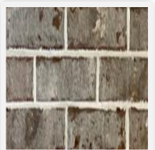
BRICK Capers Island (White Mortar with Brown Sand)
