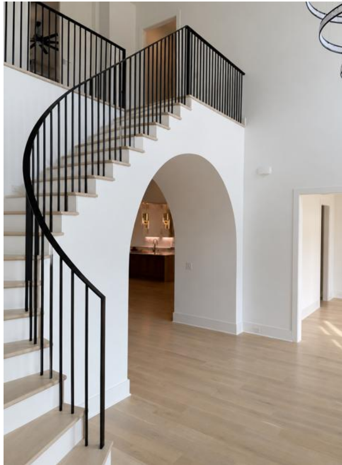
Stained Wood Treads & Painted Risers. Modern Iron Handrail & Spindles with no shoe.
